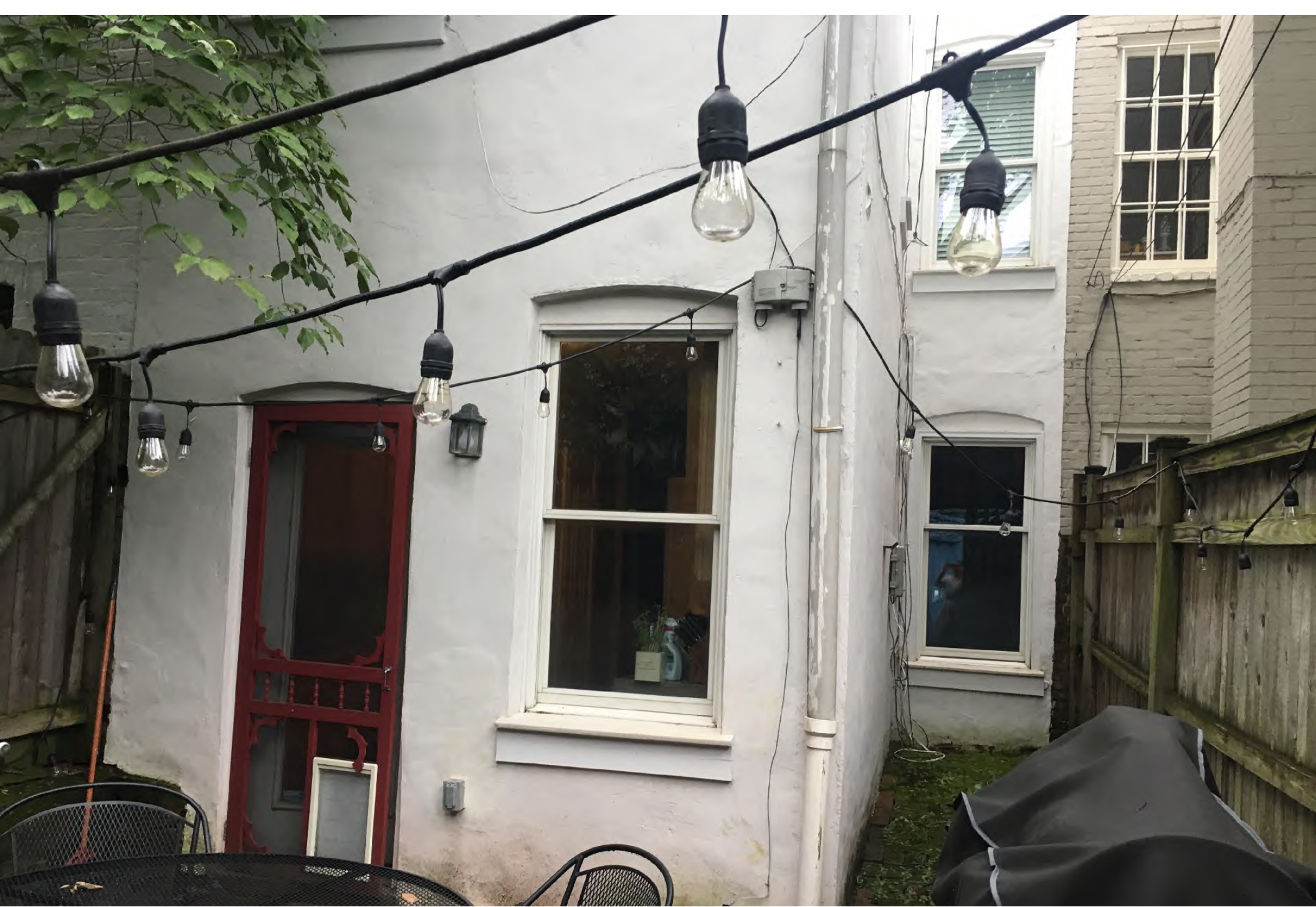
Rear View (from Patio) of 156 Duddington Place SE
