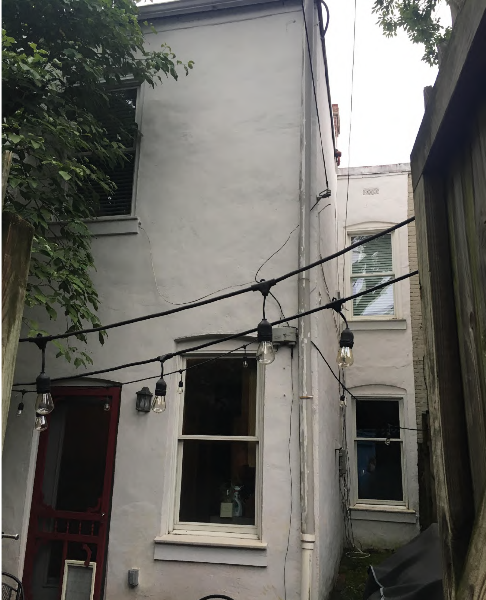
Rear View (from Patio) of 156 Duddington Place SE
