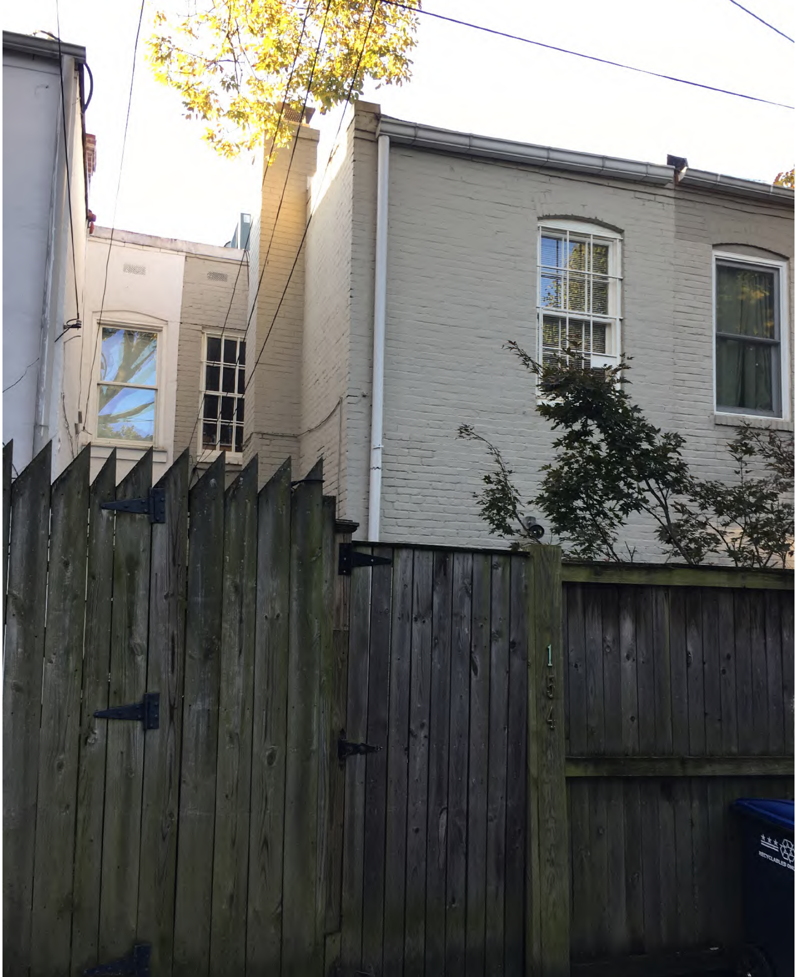
Rear View (from Alley) of Adjacent Property at 154 Duddington Place SE
