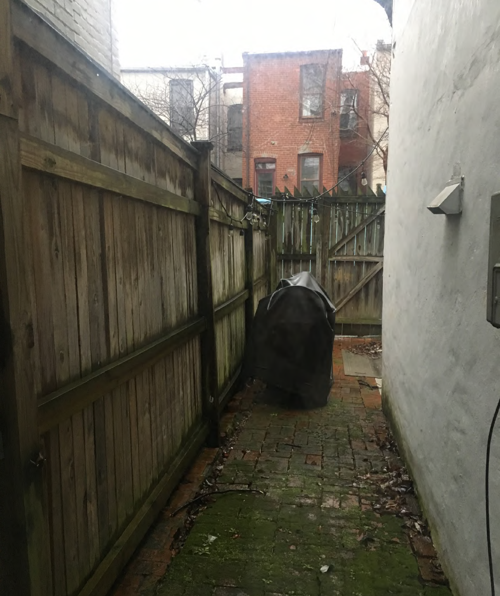
Existing Dogleg at 156 Duddington Place S.E. (View from First Story Interior)
