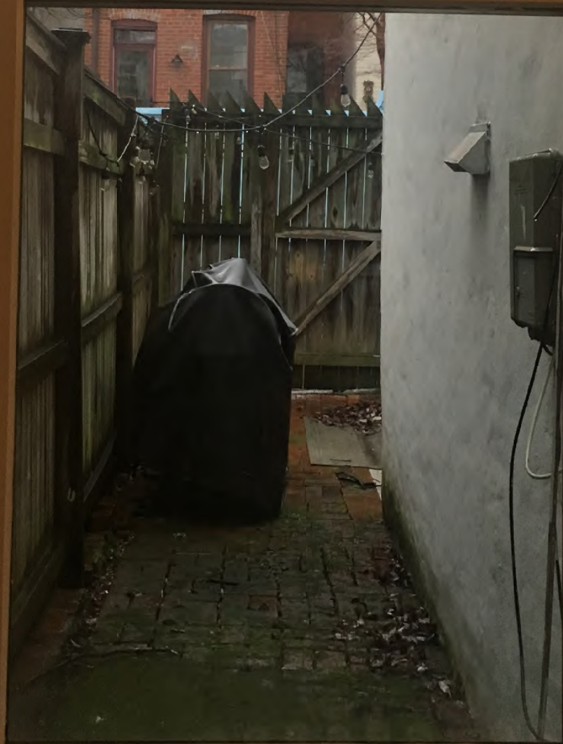
First Story Interior Looking into Existing Dogleg at 156 Duddington Place S.E.
